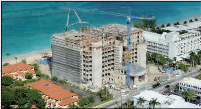
The WaterColours Condominiums under construction.
