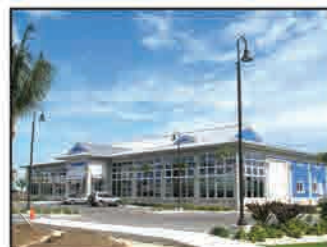
Scott's Marine Building, Barcadere
