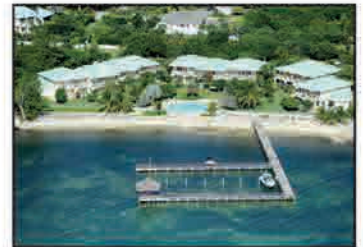
Pirate's Lair Rebuilding
