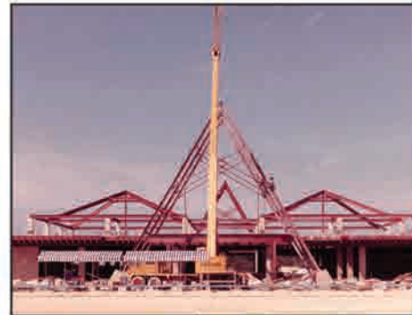
View of the Airport under construction.
