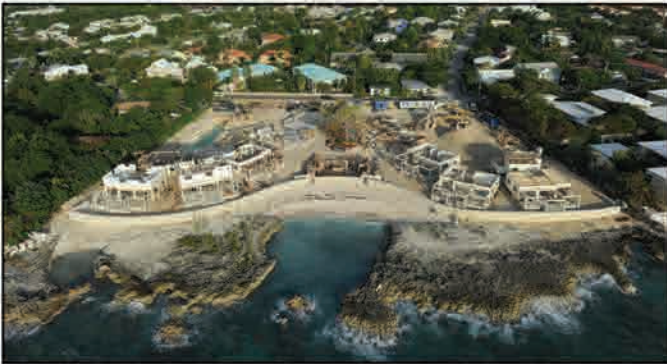
Case Luna Beachfront Villas under construction.
