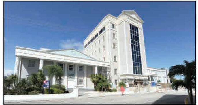
Appleby Tower under construction.
