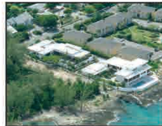
South Sound Private Residence
