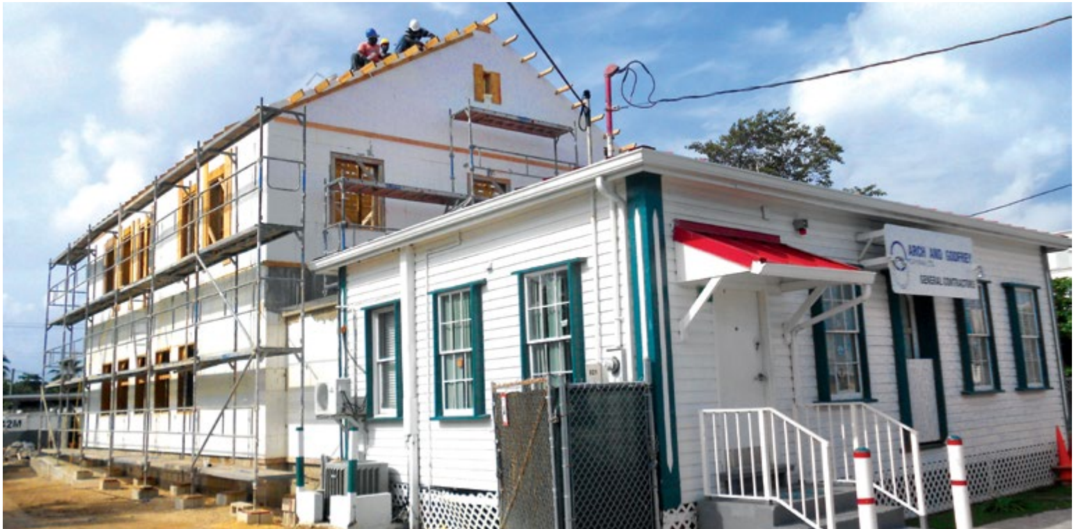
ARCH & GODFREY, HEAD OFFICE – 2021 GOVERNOR'S AWARD RECIPIENT FOR DESIGN AND CONSTRUCTION EXCELLENCE IN THE CAYMAN ISLANDS.
